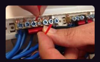
A **T1150** detector is cable tied to each neutral bar. Once all devices have been installed correctly they are wired according to the function required: early warning via an alarm, isolation of circuits or both.
