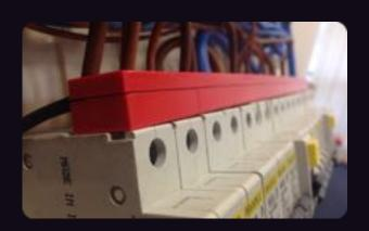
This ensures that the carriage is held in close contact with connection points on each MCB, optimising heat transfer.
