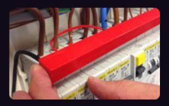
With the supply to the consumer unit isolated and front cover removed, installation is simple and straightforward. The **T11XX** carriage is held in place using the high temperature cable ties supplied to secure it to the existing wiring.
